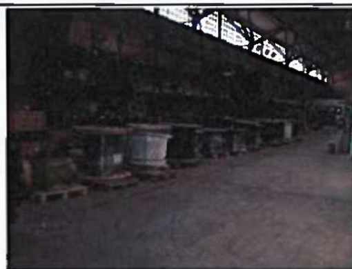
Store – storage of electric cables
